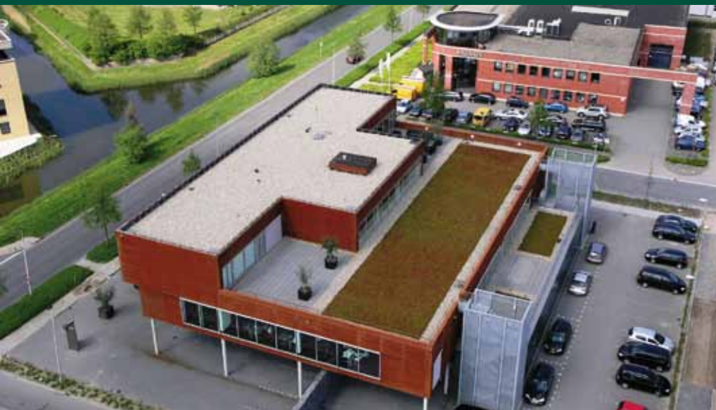
Sedumdak NSecure Barendrecht
