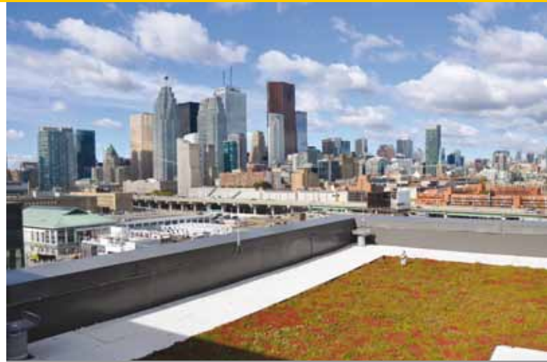
Tedco Corus Building in Toronto, Canada.
